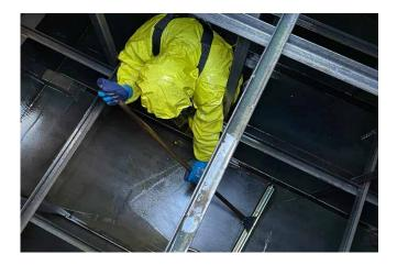
Fuel tank cleaning is essential maintenance for anybody that stores fuel. We carry out a visual inspection of the outer shell of your fuel tank to ensure that there is no damage, rust or seepage. We recommend carrying out a full cleaning and inspection of the inside every three years. This checks the integrity of your fuel storage tanks.
